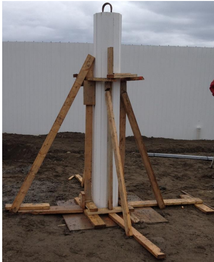
Figure 2: Typical wood bracing
